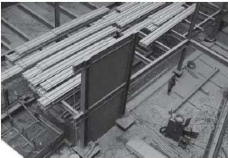
Fig. 1-34. SPW details for ICRM building (courtesy of Louis Crepeau and Jean-Benoit Ducharme, Groupe Teknika, Montreal, Canada).
