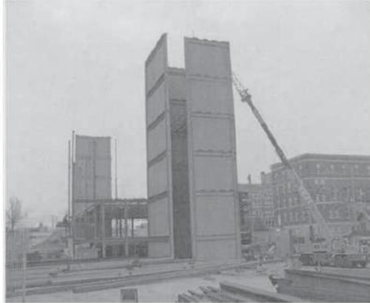
Fig. 1-31. Core wall at middle of ING building (courtesy of Louis Crepeau and Jean-Benoit Ducharme, Groupe Teknika, Montreal, Canada).
